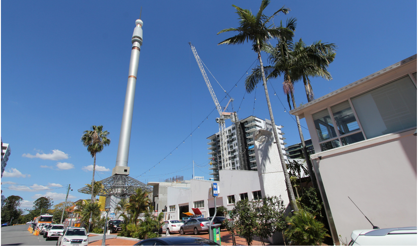
Photography: Pradella's SkyNeedle apartment project underway in West End, Brisbane.
