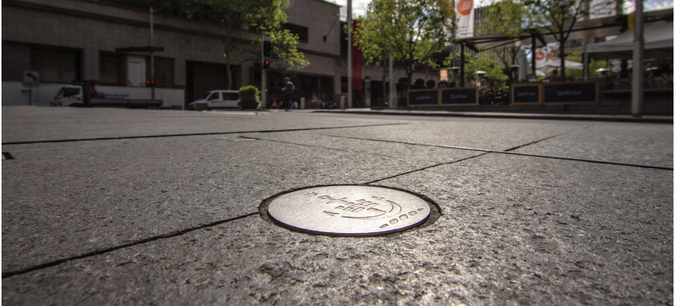
Photography: Stainless Steel Decorative Edge Covers of the type being used at New Farm Ferry Terminal upgrade.
