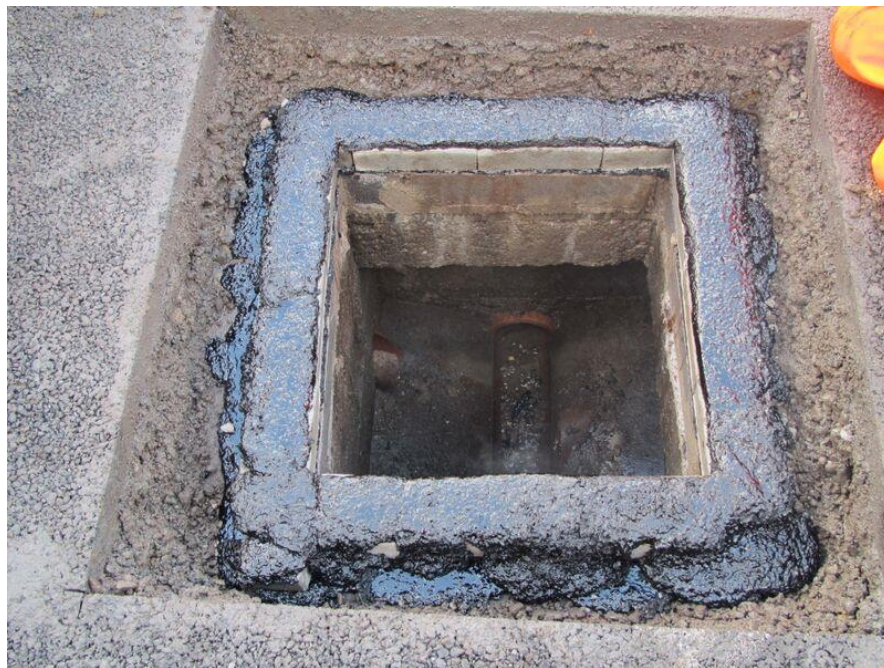
Polymer modified mastic asphalt as bedding mortar
