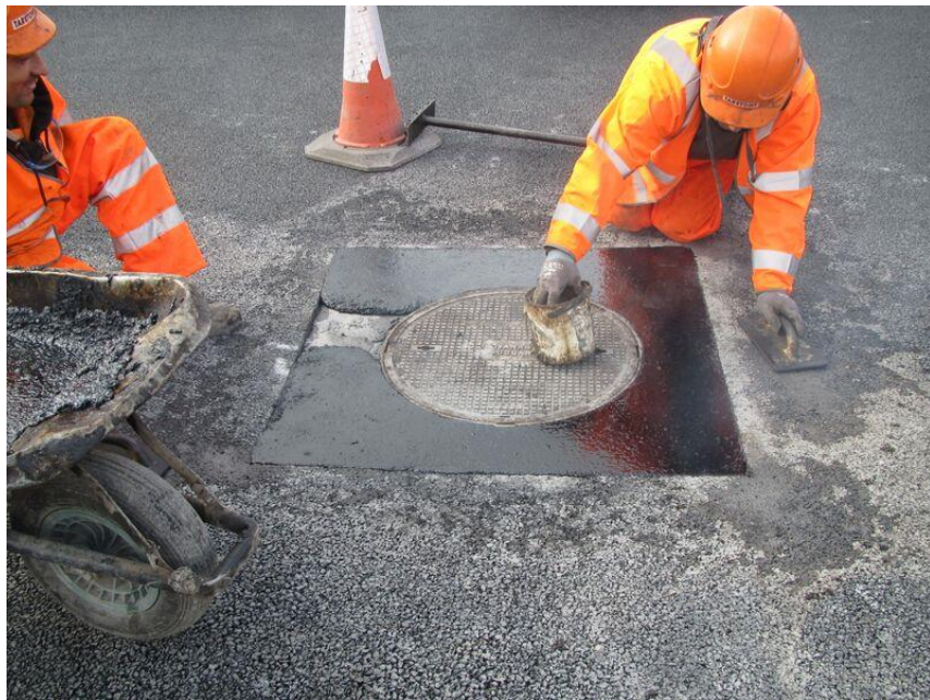
Polymer modified mastic asphalt placed as surface course
