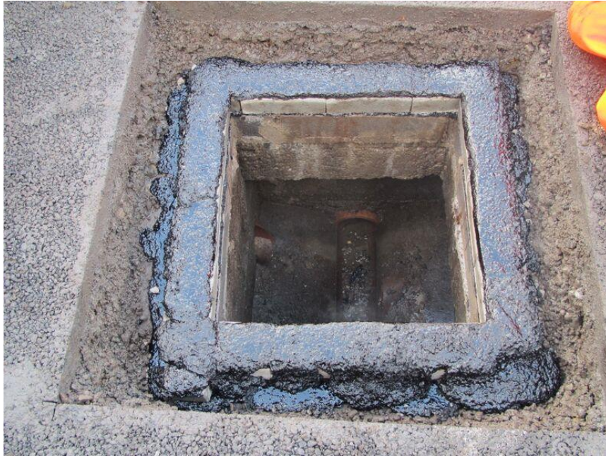
Second layer of polymer modified mastic asphalt as bedding
