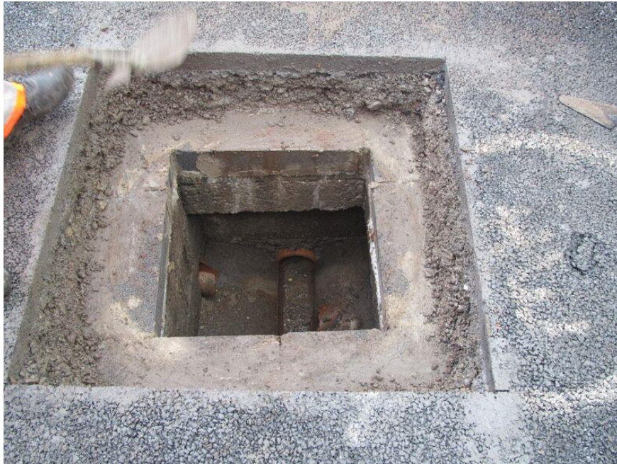
Manhole chamber top exposed
