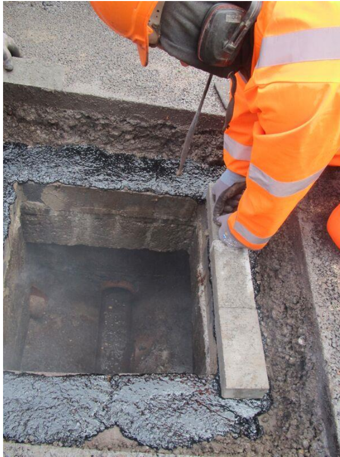
Layer of engineering brick
