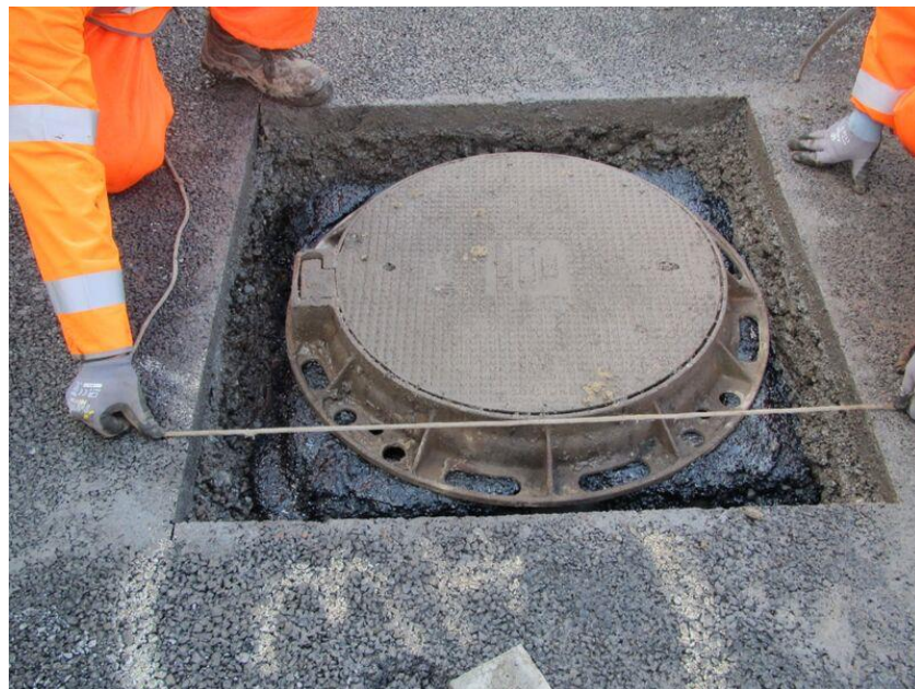
Placing frame and cover
