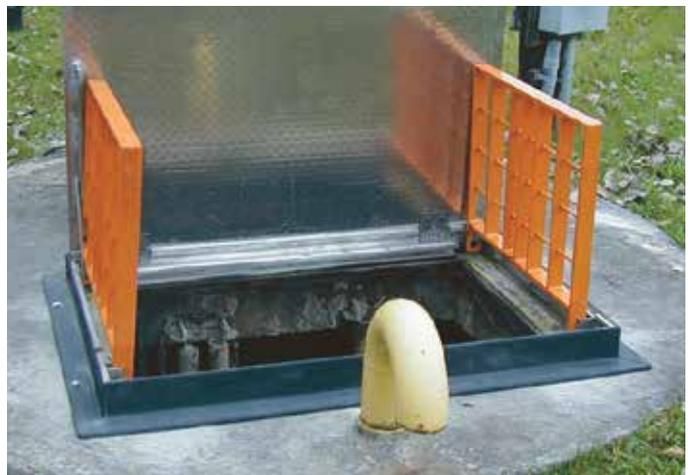
Open safety grates: Safety orange painted aluminium grates provide a visual barrier around pit.
