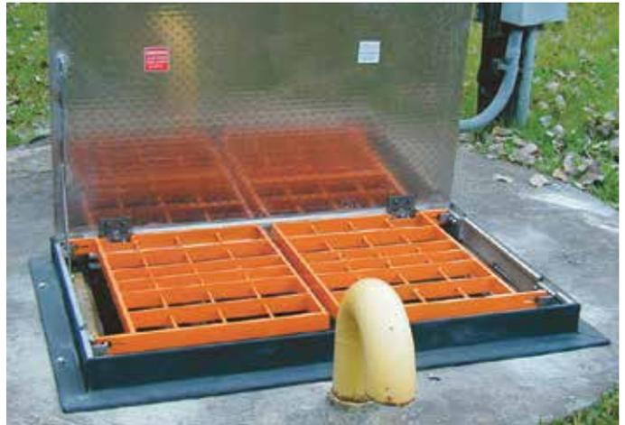
Closed safety grates: Safety orange painted aluminium grates provide 14.36 kPa non-traffic pedestrian rated fall through protection.
